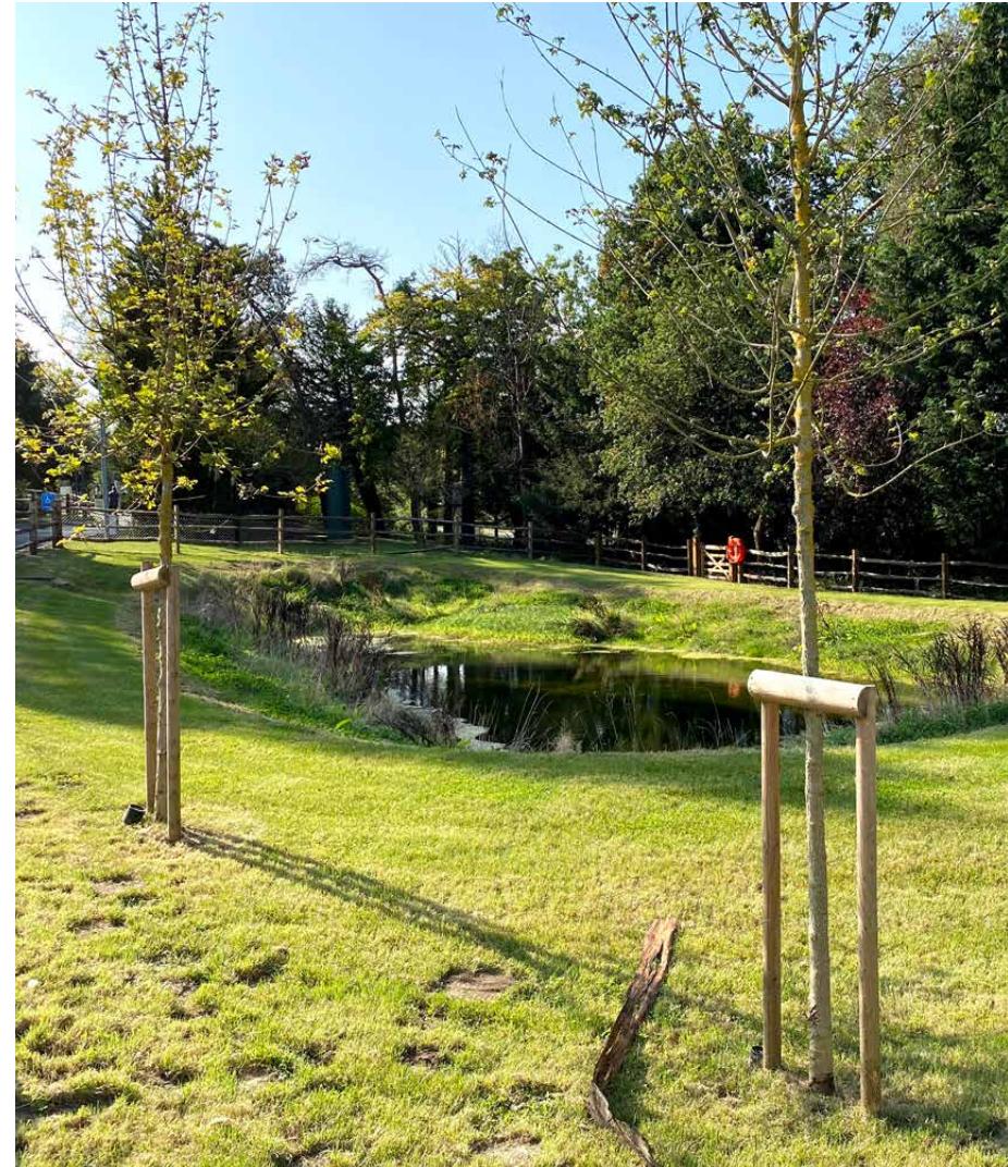
Landscaped attenuation basin
